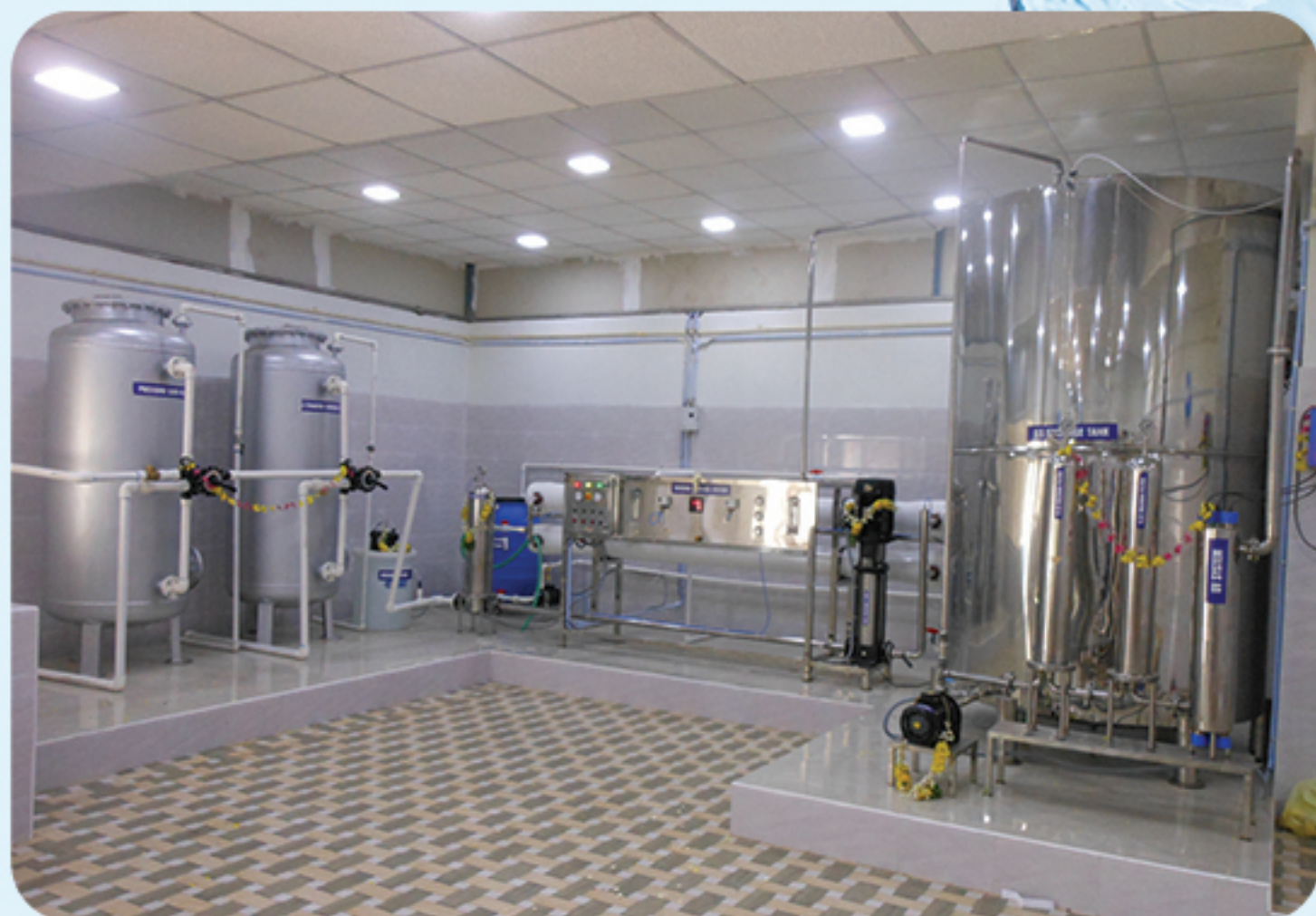
6000LPH (Membrane filtration System with storage tank, Post filtration, UV and Ozone Generator Disinfection System)
