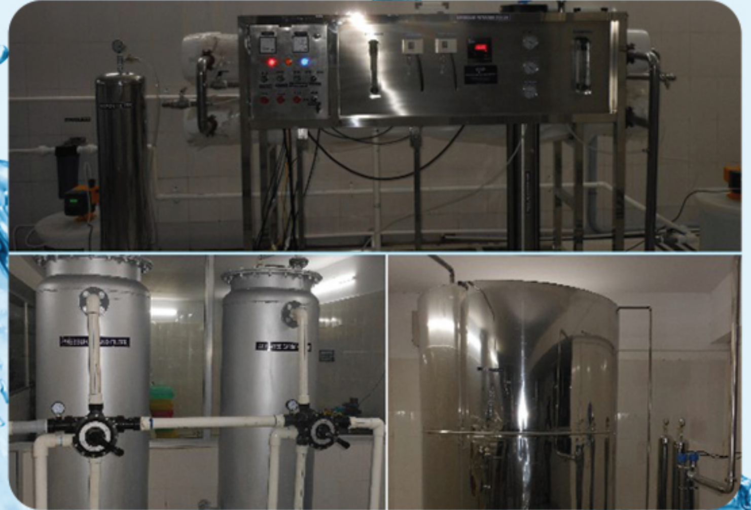
4000LPH (Membrane filtration System with storage tank, Post filtration, UV and Ozone Generator Disinfection System)
