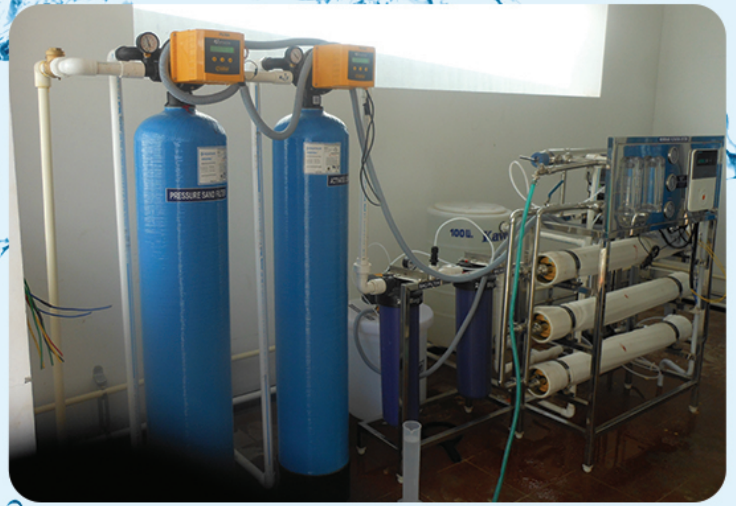
600LPH (Automatic operated membrane filtration and UV disinfection system with SS 304 pipelines)
