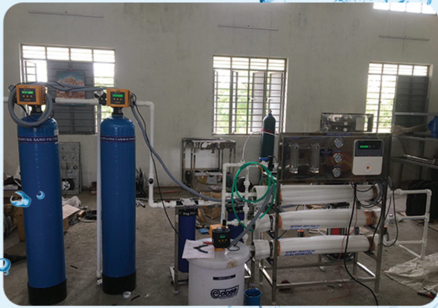
600LPH Fully automatic membrane filtration (UPVC Pipeline)
