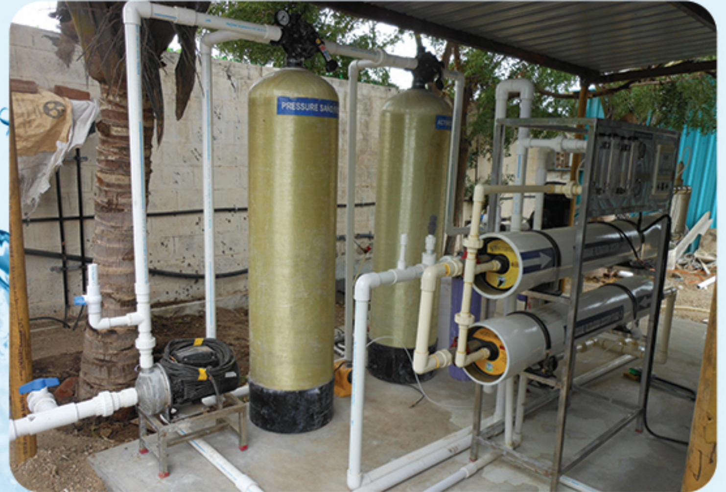
2000LPH (Membrane filtration system with Pressure sand filter, Activated carbon filter, Bag filter, Micron filter 1, Micron filter 2 with Membrane cleaning and flushing system)
