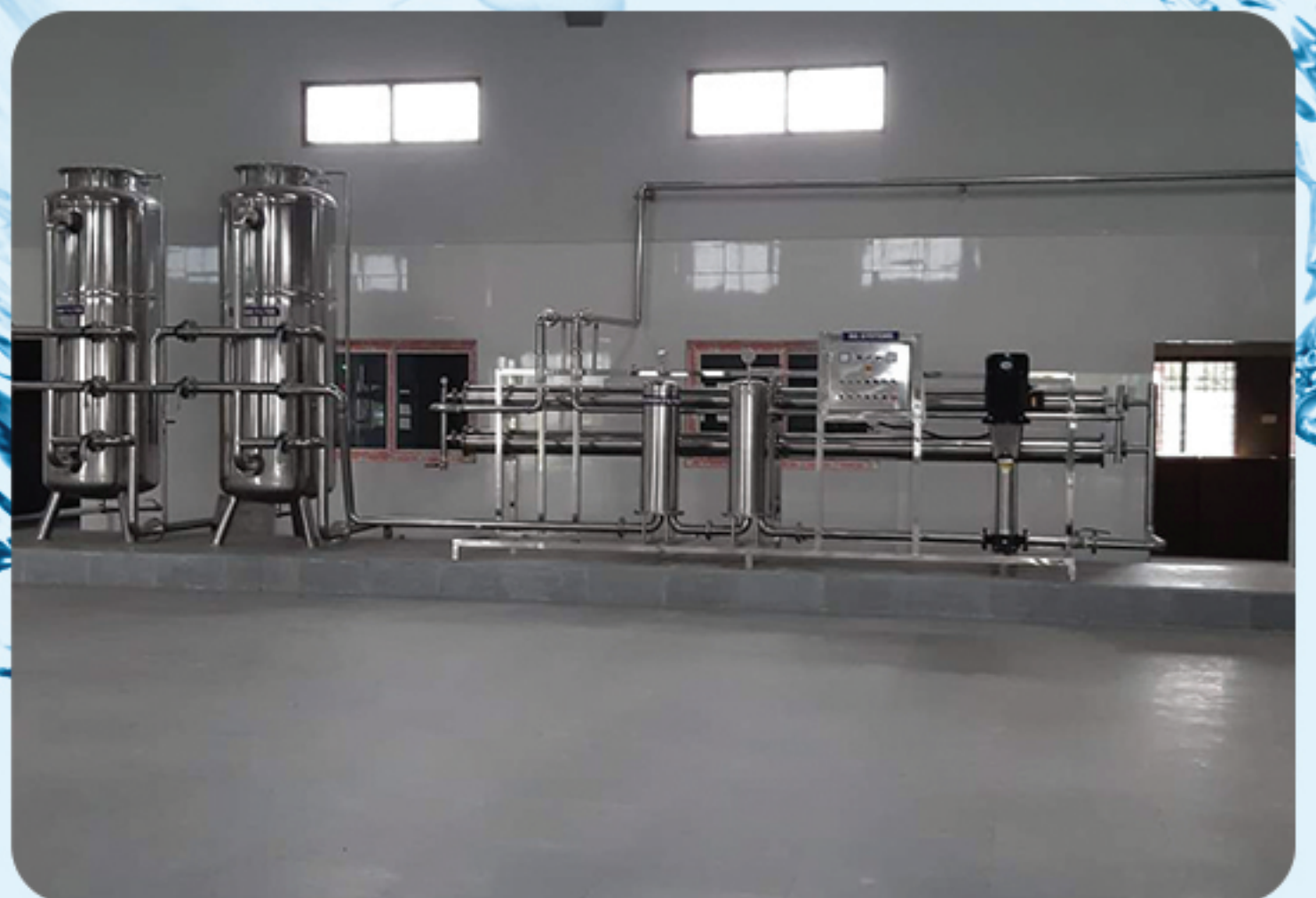
10000LPH (Fully SS304 membrane filtration system)
