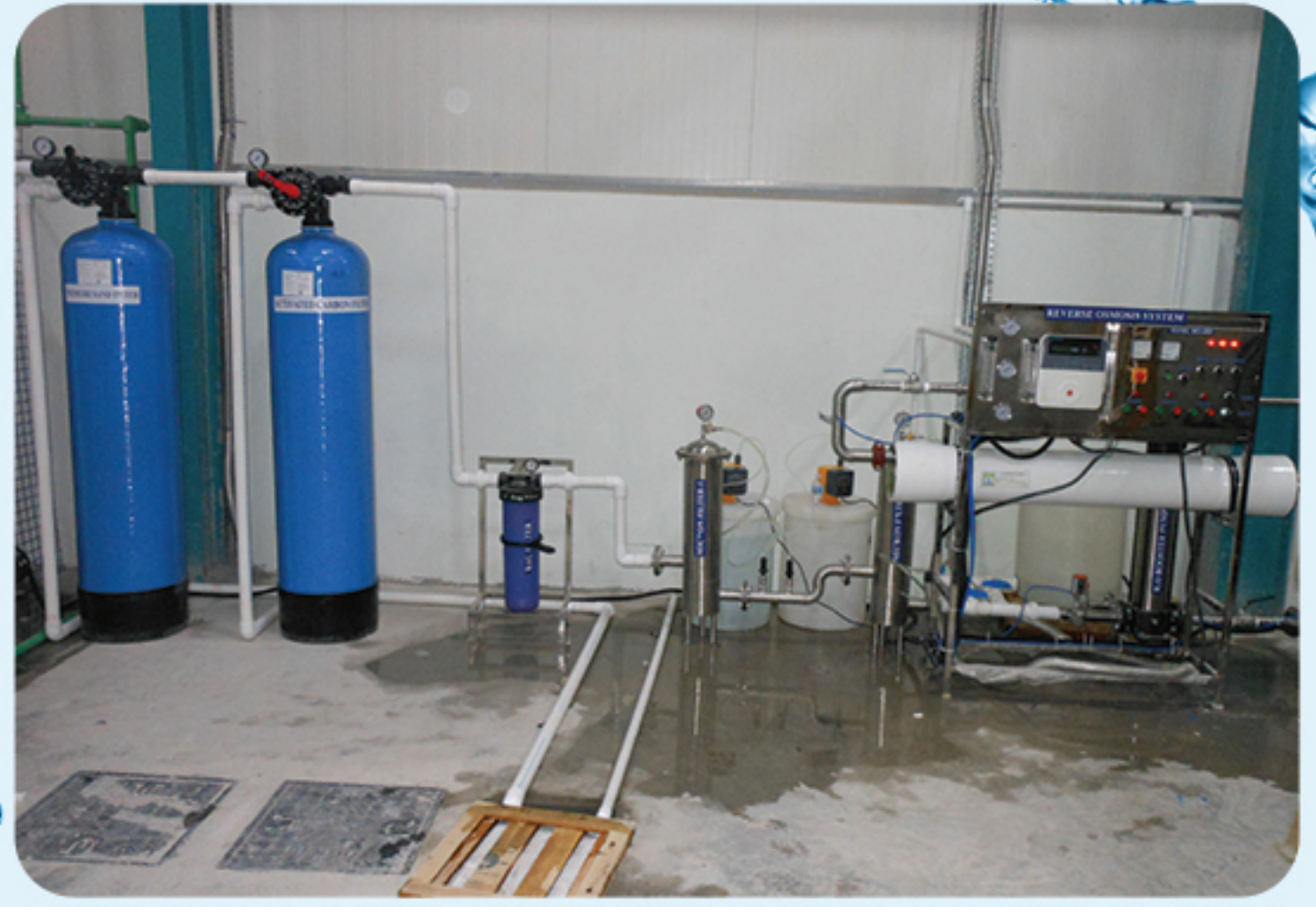
1000LPH (Pressure sand filter, Activated carbon filter, Bag filter, SS Micron filter 1, SS Micron filter 2 with RO system and RO cleaning and flushing system)
